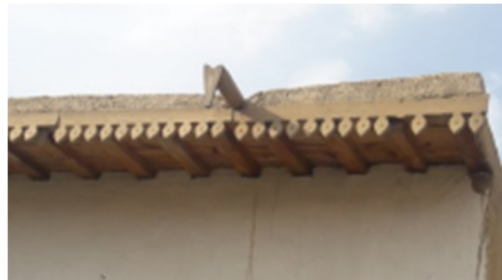
Figure 14. Gargoyle on the roof (Uşma, Urfalıoğlu, 2018)
