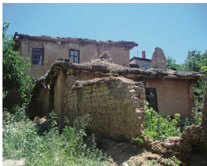
Figure 3. Masonry system (Karakul, 2011)
