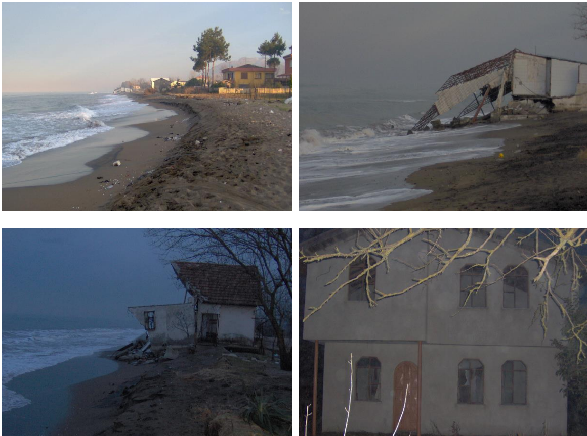
Figure 6. Destructions in real estates in the coastal zone (Ülger 2006)
